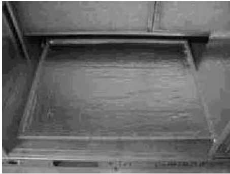
Figure 17: Return Downflow Plenum With Panel
