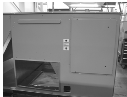
Figure 15: Side panels with hole plugs
