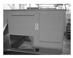
Figure 17: Side panels with hole plugs
