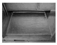
Figure 18: Return down flow plenum with panel
