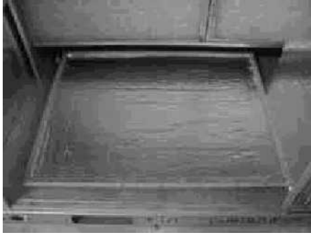
Figure 17: Return Downflow Plenum With Panel
