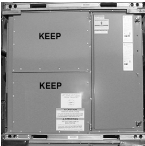
Figure 19: Save Side Panels For Economizer Hood Tops
