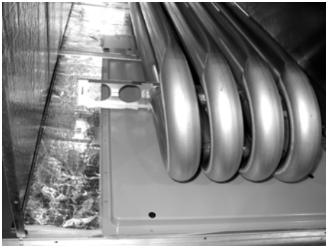
Figure 18: Discharge Panel In Place
