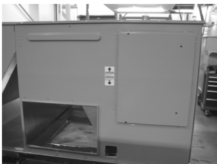
Figure 18: Side panels with hole plugs
