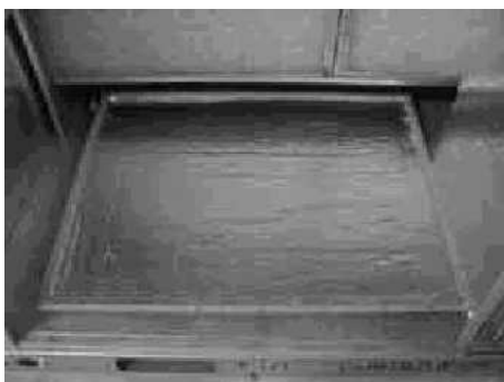
Figure 19: Return downflow plenum with panel
