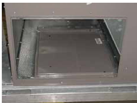
Figure 20: Discharge panel in place
