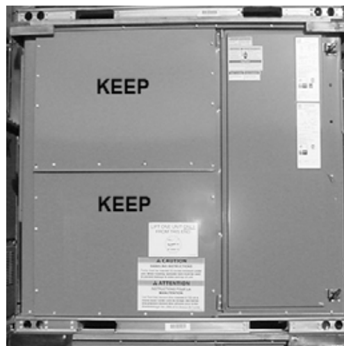
Figure 21: Side panels for economizer hood tops
