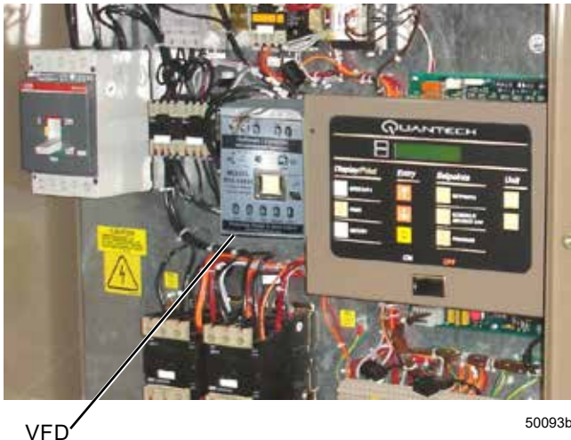
FIGURE 45 - TYPICAL VFD LOCATION
