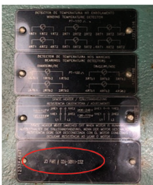
Example WEG aux. motor nameplates (JCI part number circled)
