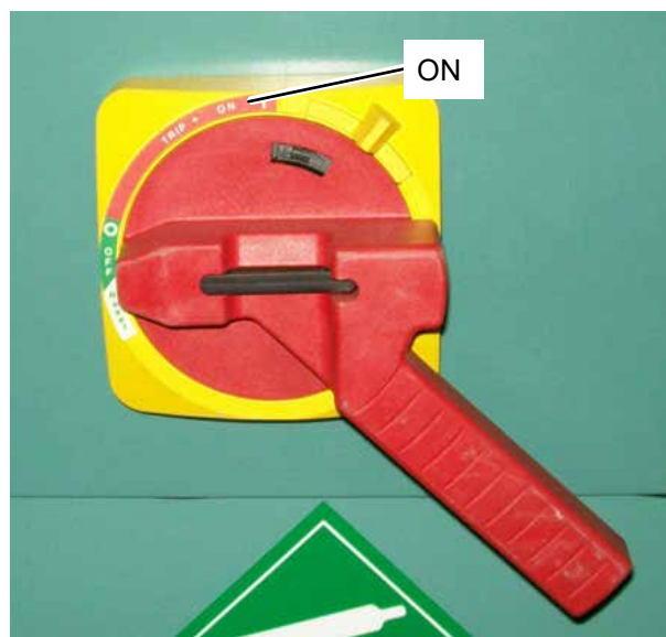
FIGURE 1 - EMERGENCY SHUTDOWN HANDLE
