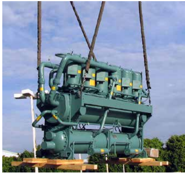
FIGURE 8 - CHILLER RIGGING AND LIFTING WEIGHTS
